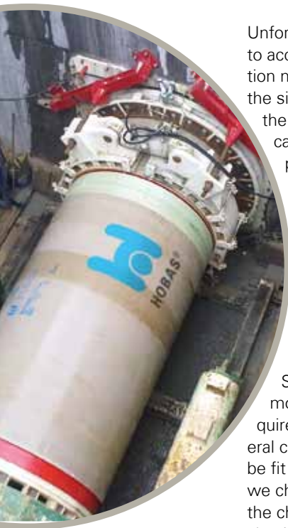
HOBAS Pressure Pipe Jacking under the Lido of Venice, IT
